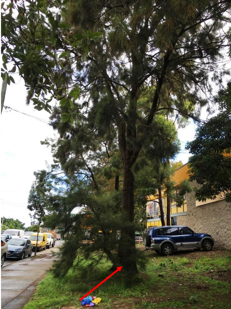
Photo 7 – Tree HV72 (noted with red arrow). Tree requires removal to accommodate proposed works.
