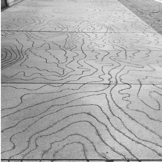
Figure 9. Granite footpath showing topographical layers (Source: Pinterest – Styraciflua).
