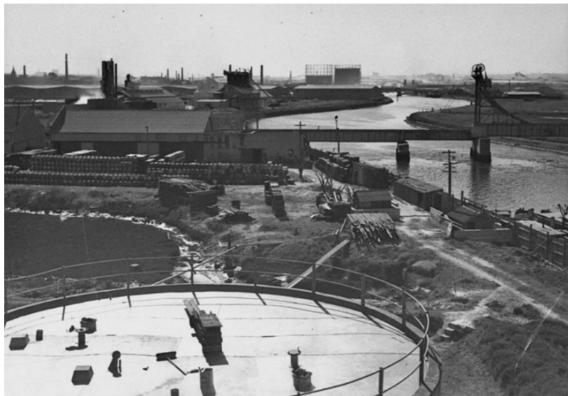
Figure 15. View of Lifting Span Railway Bridge across Alexandra Canal (Source: 'H.C Sleigh's Shea's Creek Depot, Alexandria', State Library of NSW, call no.20943).
