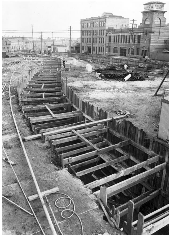
Figure 19. Formwork for construction of underground stormwater channel feeding into the Alexandra Canal, Waterloo 3 August 1928 (Contributed By City of Sydney Archives [67311] (Sydney Water 'A' Series Photographs A546)
