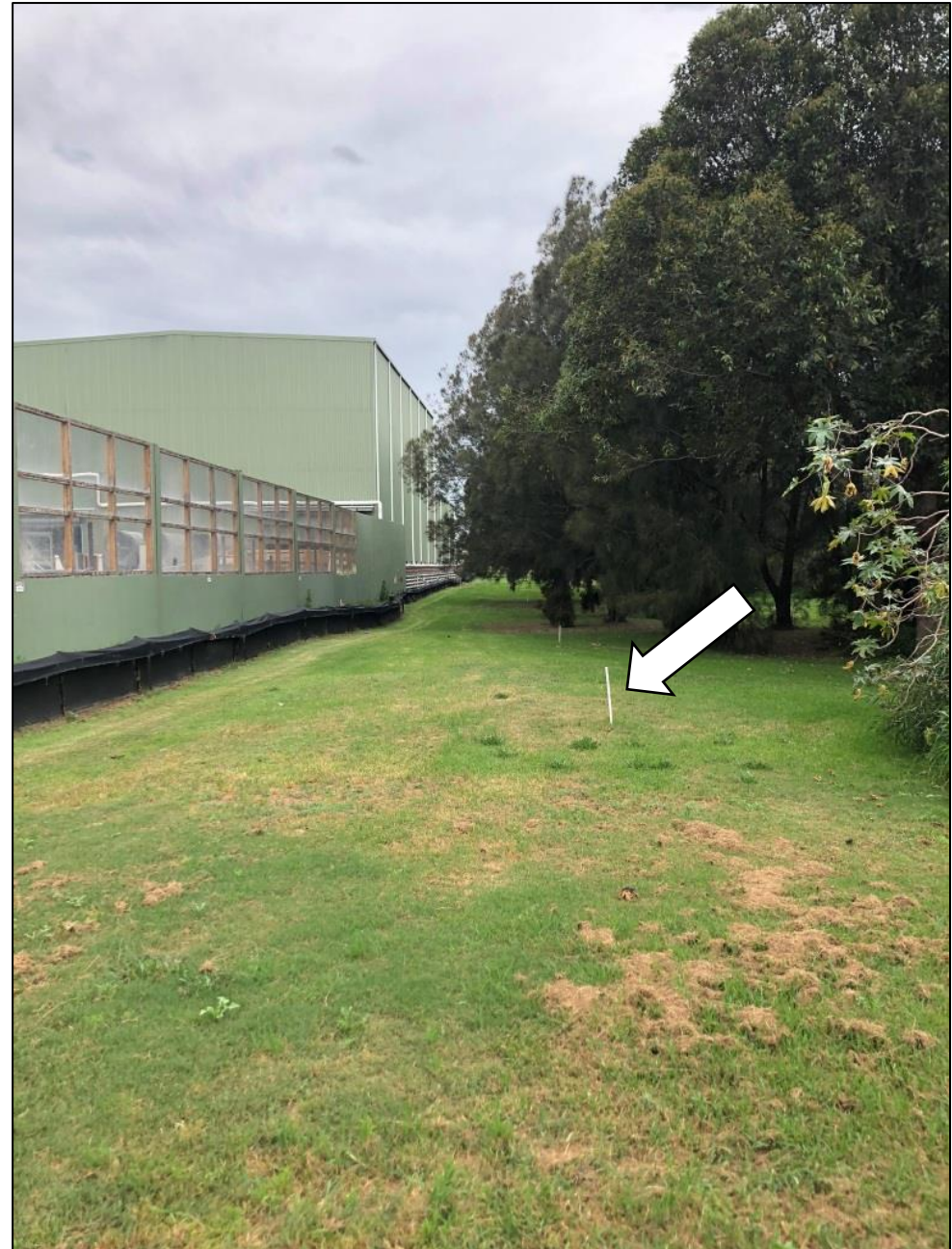
Plate 4 – Overview of site, green Hoarding (with clear sections for light filtration) can be noted to left of photo, arrow notes white marker in location of proposed realignment of Hoarding.
