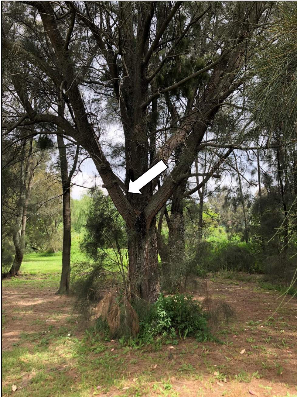
Plate 3 – Arrow notes to large diameter limb on T13 that requires removal to allow Hoarding realignment.
