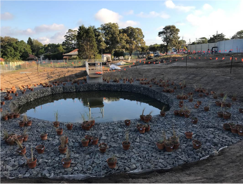
Figure 3: Gabion ring wall around Pond 3, 20 April 2018.
