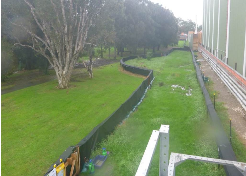
Figure 1: Relocated Fence on Southern side of compound
