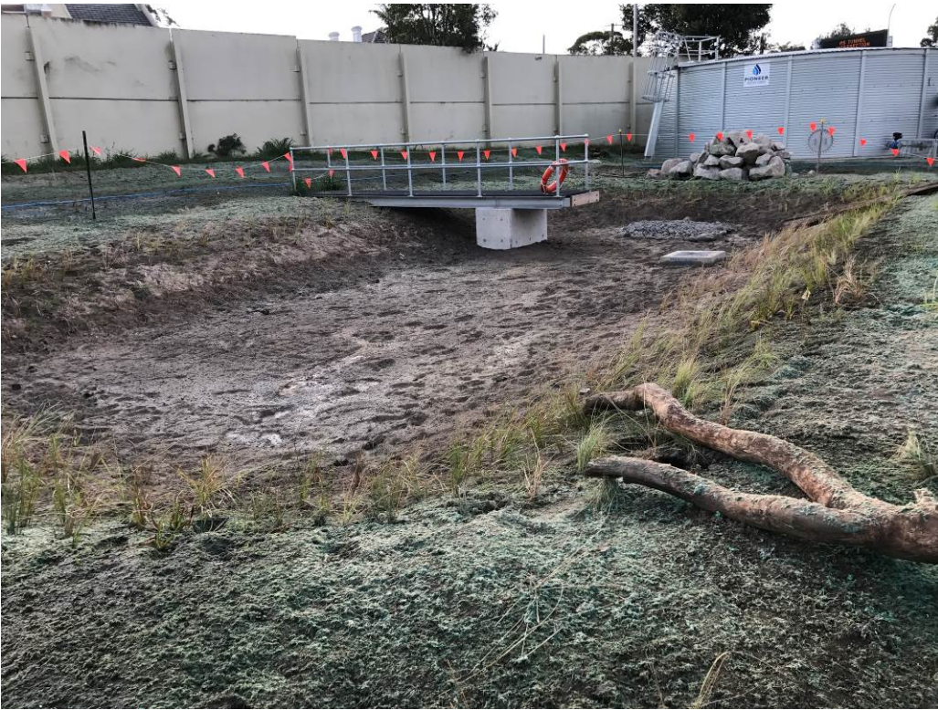
Figure 4: Pond 1 prior to refilling, 26 April 2018
