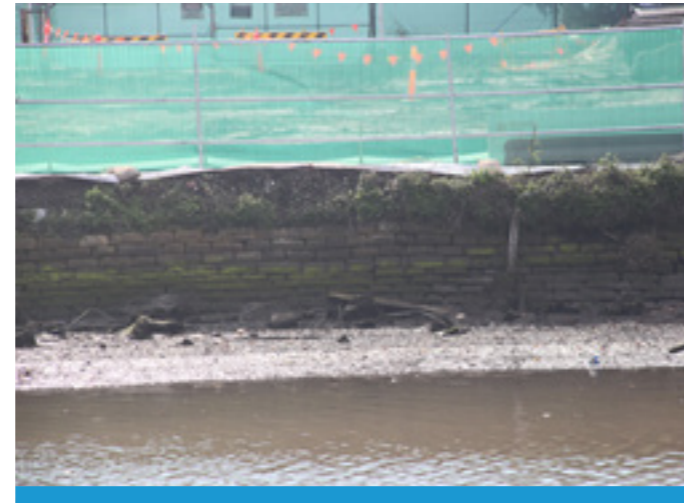
Figure E-19 - Section of western wall in the location of Bridge 10
