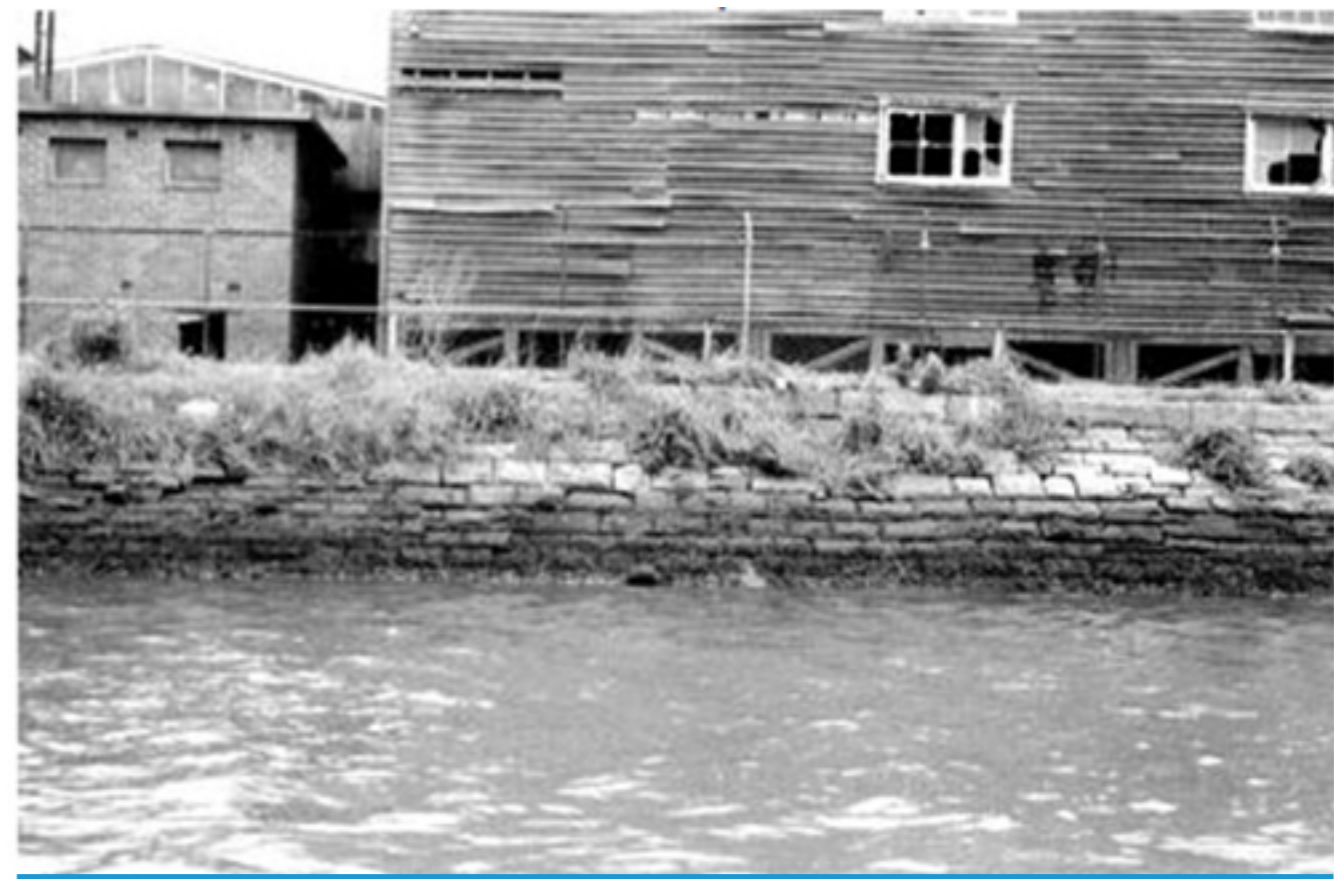
Figure E-29 - 1984 view of abandoned Wool Sheds along Alexandra Canal. Source: Graeme Andrews 'Working Harbour' Collection: 80134. GKA. City of Sydney Archives, file no. 080/080134
