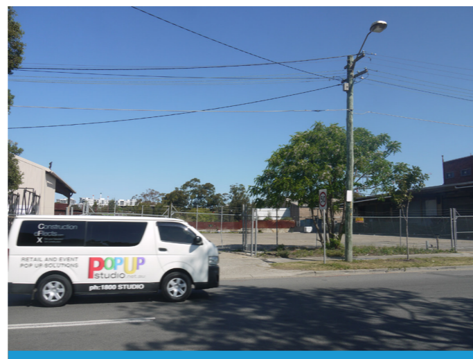
Figure E-15 - This open yard will form the main approach to the Campbell Street/Road bridge. This lines up with the eastern approach on the opposite bank and the proposed alignment into Campbell Street/Road.
