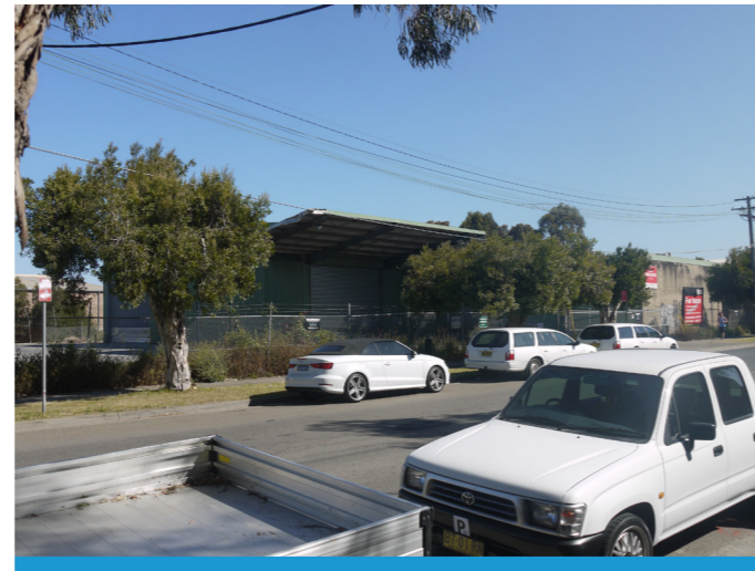
Figure E-3 - The western approach to the Gardeners Road bridge. The area is heavily developed in terms of industrial factories and warehouses. The approach makes use of existing open yards, but will require the demolition of factories and warehouses which are of little significance.
