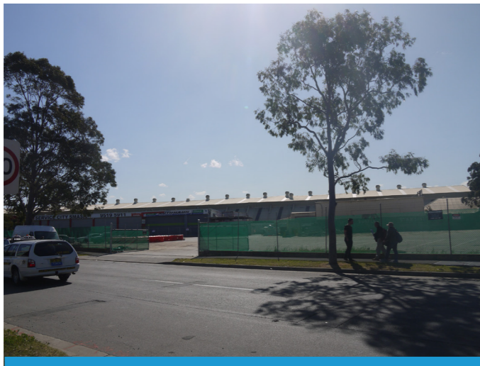
Figure E-2 - The western approach of the Campbell Street/Road bridge. The building in the background is Rudders Bond, which has been approved for demolition as a part of the SSL. The approach to the bridge will make use of the open yard and the space provided through the demolition of Rudders Bond.
