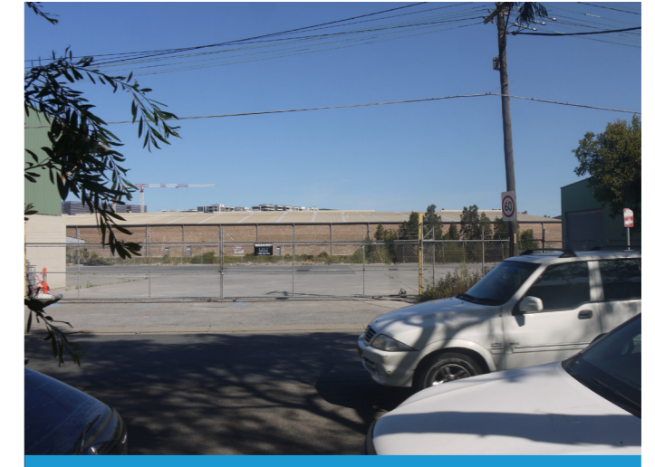
Figure E-5 - This large open yard provides the approach for the Gardeners Road bridge. The structure in the background is the State Archives building.
