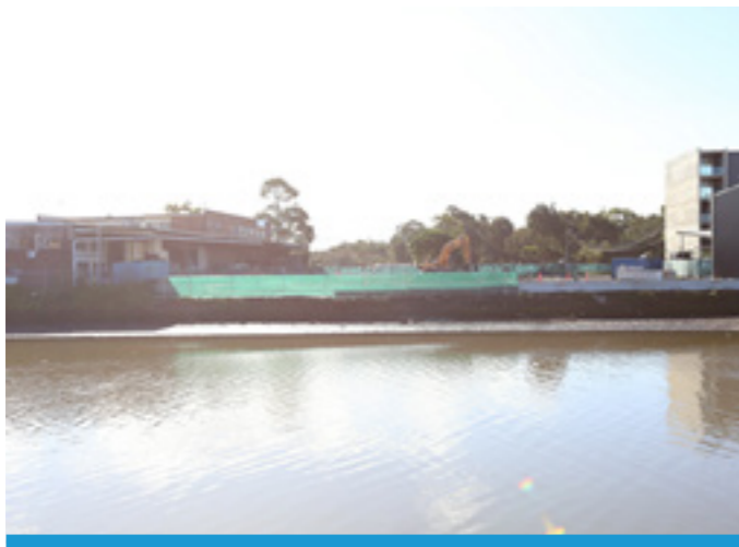
Figure E-20 - Western wall in the location of Bridge 10.
