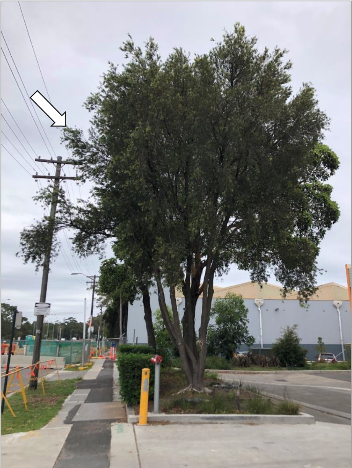
Plate 7 – A3 29 – Weeping Bottlebrush – Arrow notes limbs requiring removal to accommodate light pole installation/positioning.
