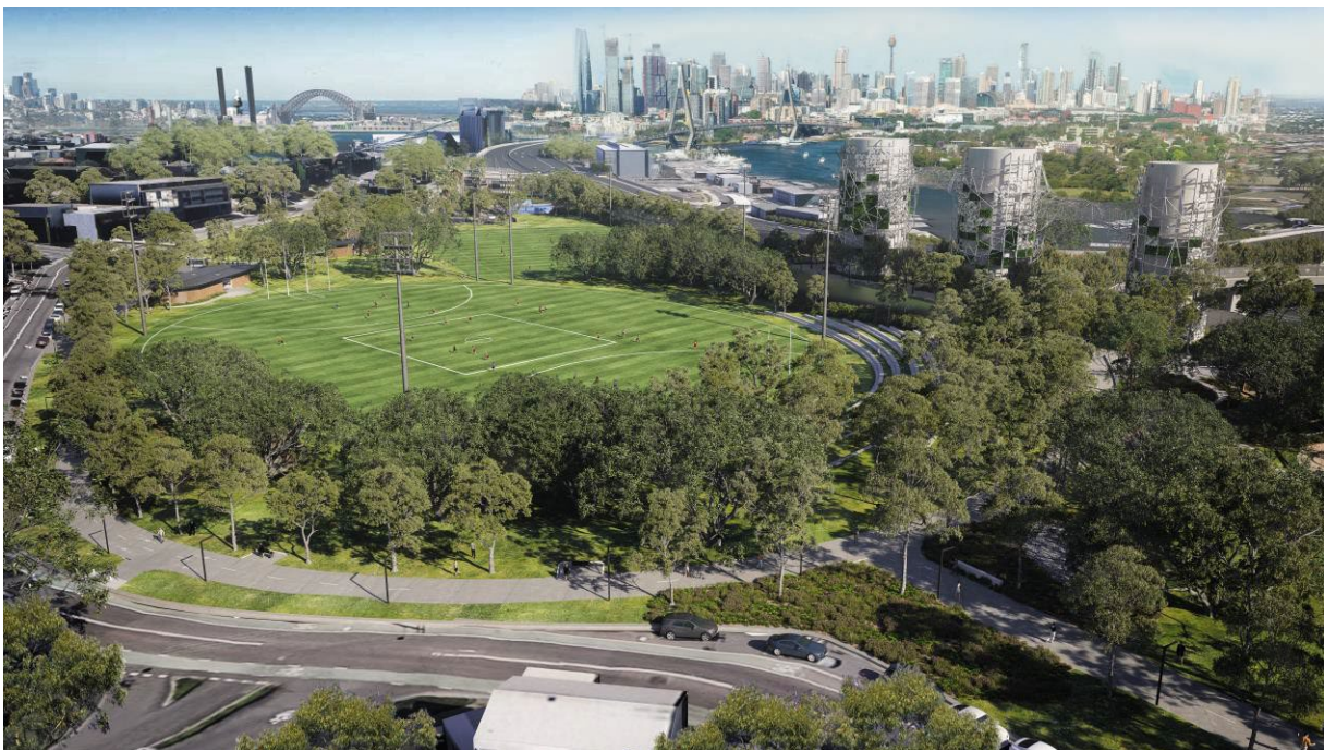
Figure 1: Rozelle Parklands two sports fields and facilities building
