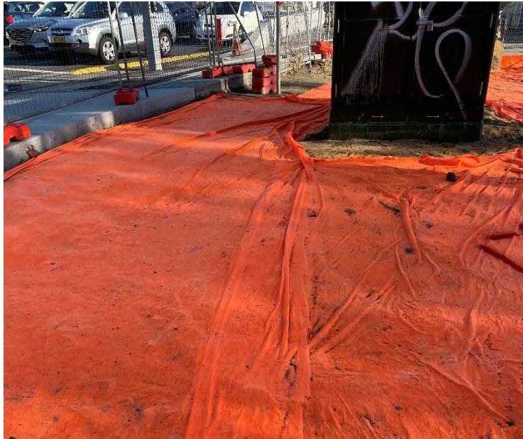
Figure 5.2 Geotextile marker layer
