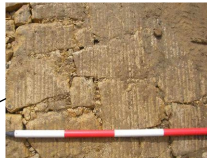
Figure 2: Close up detail of the sandstone surface showing material type, formation and construction detail. This is essential for establishing date of the feature.
