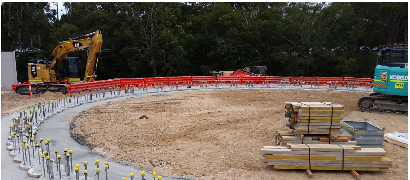
Concrete pouring around the shaft at the Bexley south compound to form the base of the spoil shed, January 2017
