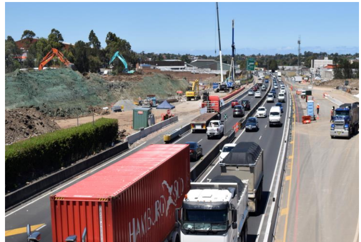
Work underway to build the New M5 tunnel portals, November 2016
