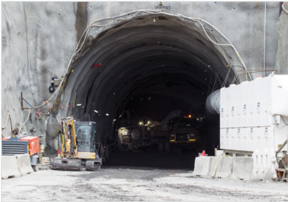
Progress of St Peters New M5 tunnel, February 2017
